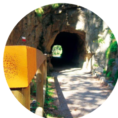
Tunnel on the Matxos path
