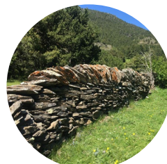
Dry stone wall
