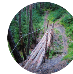
Bridge across the path
